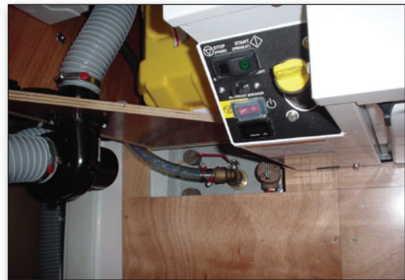
Seacock Access. The seacock and local generator controls are easily accessible.
