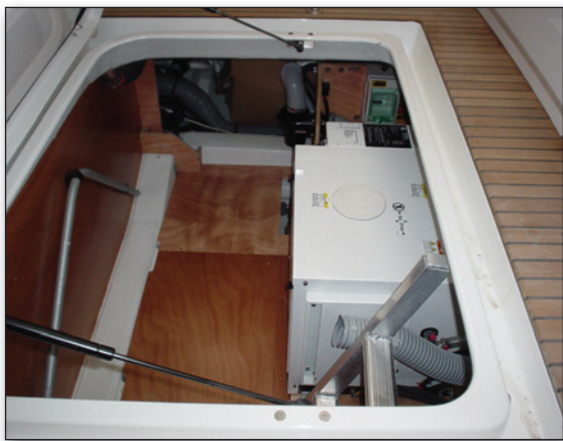
The MDKBJ unit installed in the lazarette of The Greatest Loop. Plenty of room for service access.
